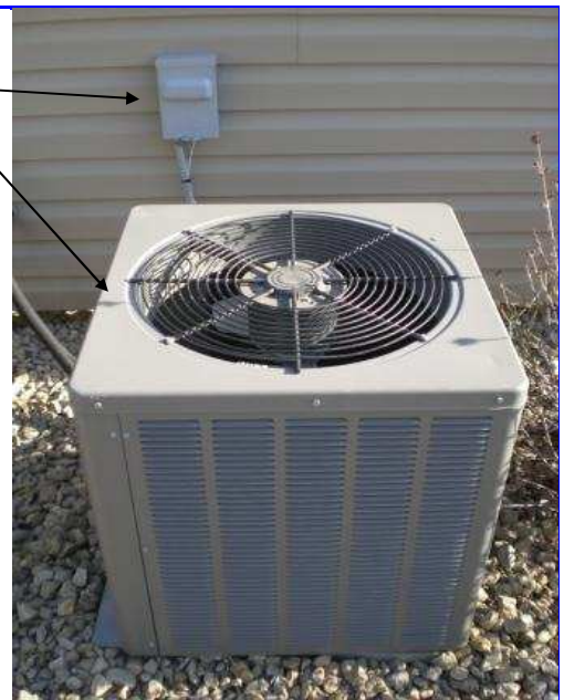
AC condenser cabinet and disconnect
